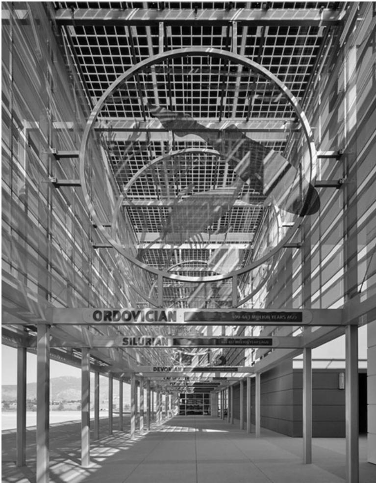
**Figure 5.12** Paleontology Museum building integrated photovoltaic (BIPV) solar power system. *Photo courtesy of Lehrer+Gangji architects.*
