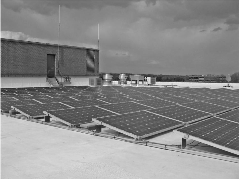
**Figure 3.68** Nonpenetrating roof-mounted solar power installation with adjustable tilt support platform. *Photo courtesy of DPW Solar.*
