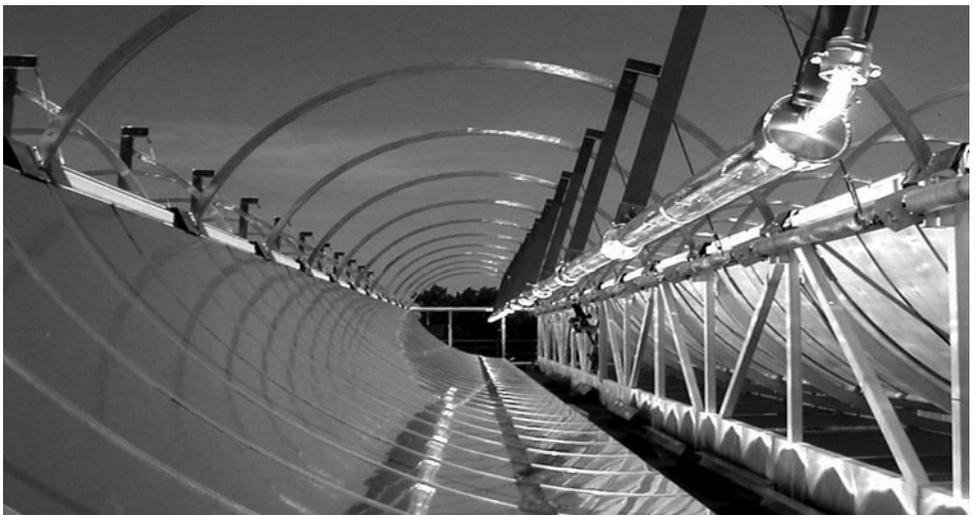
**Figure 6.9** Passive parabolic concentrator installation. *Courtesy of Solargenix.*
