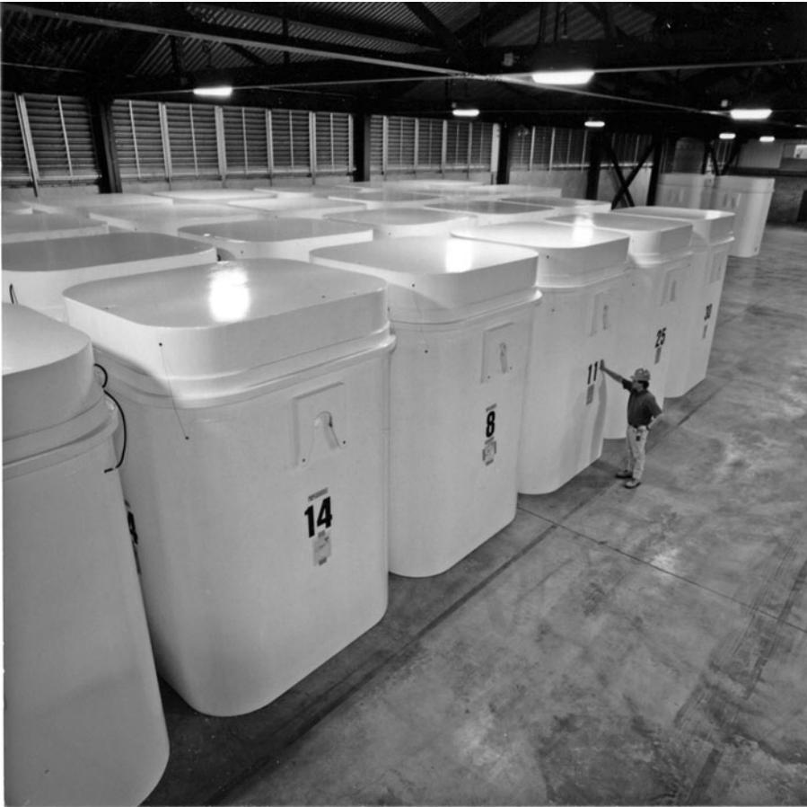
**Figure 13.8** CANDU reactor used-fuel container. *Courtesy of CAEL.*
