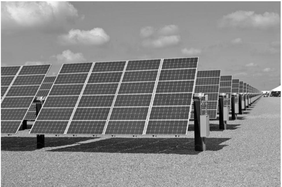
**Figure 3.71** A large-scale single-axis solar farming system, Semitropic Water District, Wasco, California. *Photo courtesy of SolarWorld.*
