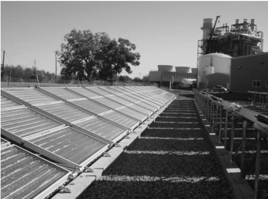
**Figure 6.7** An industrial solar water-heating panel installation.
