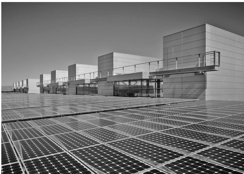
**Figure 3.67** Water and Life Museum rooftop solar power system. *Photo courtesy of Vector Delta Design Group, Inc.*
