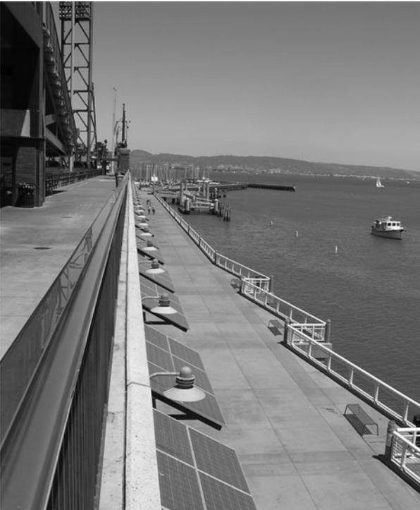
**Figure B.13** Solar power window canopy. *Photo courtesy of DWP Solar.*
