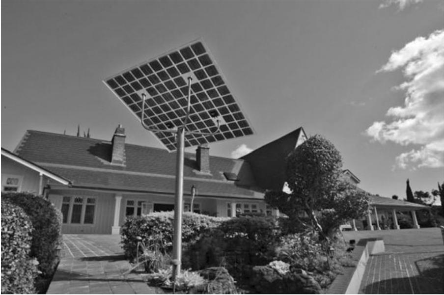
**Figure B.8** Building-integrated solar power stand. *Photo courtesy of DWP Solar.*
